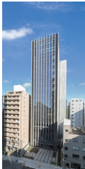
Promoted energy-saving initiatives, including switching to LED lighting at each workplace
