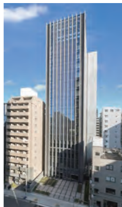
Promoted energy-saving initiatives, including switching to LED lighting at each workplace
