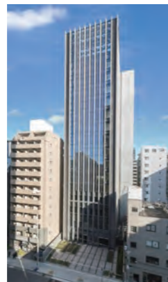
Promoted energy-saving initiatives, including switching to LED lighting at each workplace
